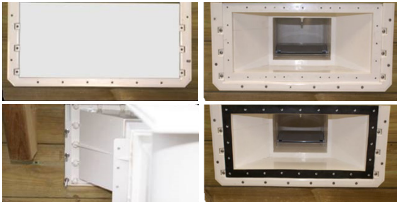
Figure 24 – Montage du skimmer
