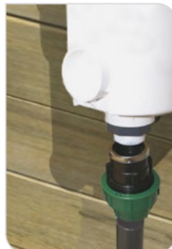
Figure 44 – Descente sous skimmer
