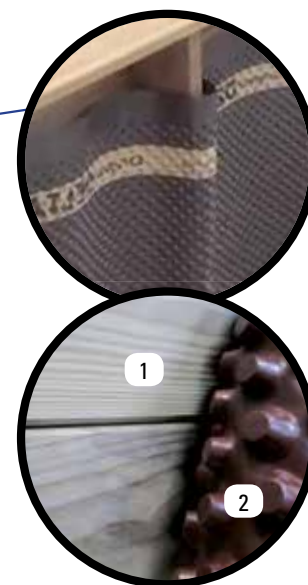
1- Wood frame 2- Roll of alveolar protection and drainage of HDPE
